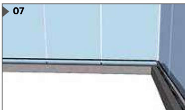
Fixed the inside system cover on the innerface of the blocks.
